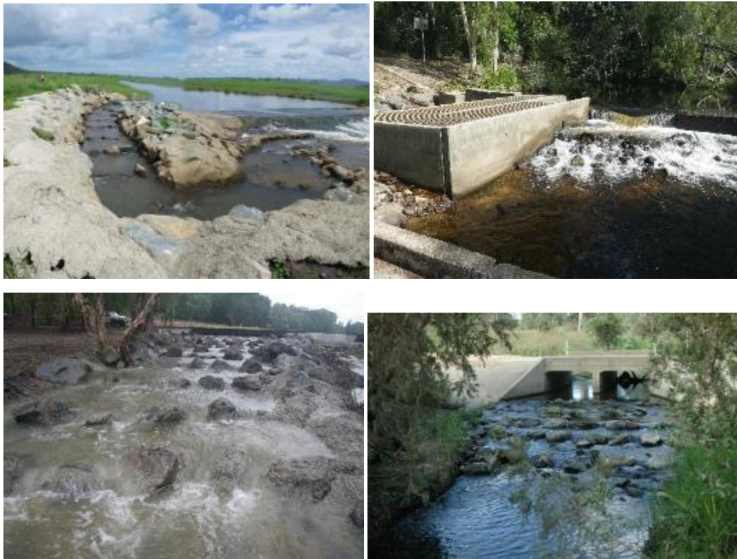
Figure 1. Four fishways constructed in the FBA Region. A) Amity Creek rock ramp fishway (top left), b) Water Park Creek vertical slot fishway (top right), c) Moores Creek rock ramp fishway (bottom left) and d) Raglan Creek rock ramp fishway (bottom right).
