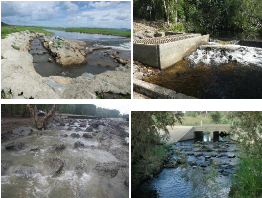
Figure 1. Four fishways constructed in the FBA Region. A) Amity Ck rock ramp fishway (top left), b) Waterpark Ck vertical slot fishway (top right), c) Moores Ck rock ramp fishway (bottom left) and d) Raglan Ck rock ramp fishway (bottom right).
