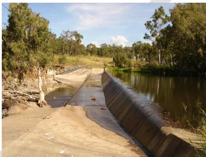
Figure 4.1. St Lawrence Weir (Barrier ID 9393) on St Lawrence Creek is a high priority barrier to fish passage within the FBA region.
